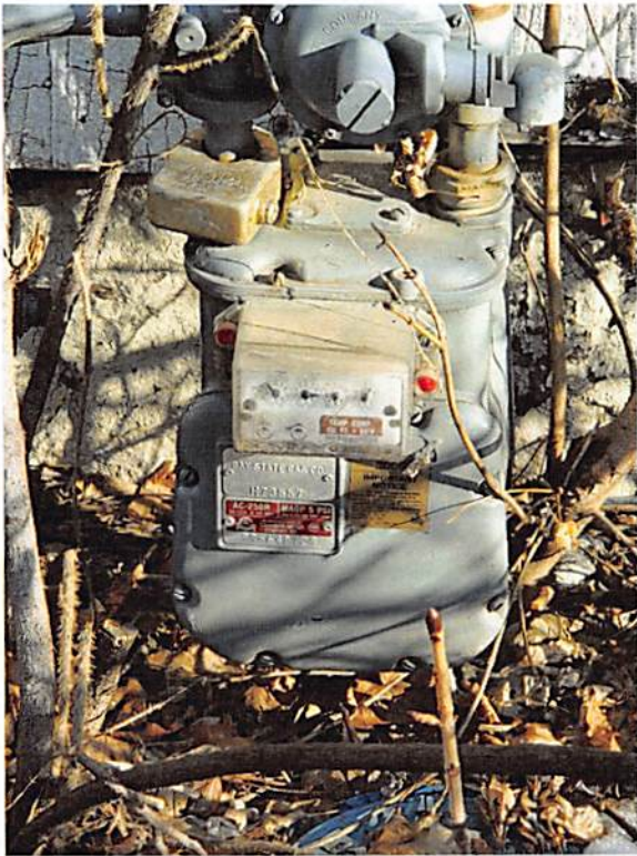
Gas service shut down and locked out.
