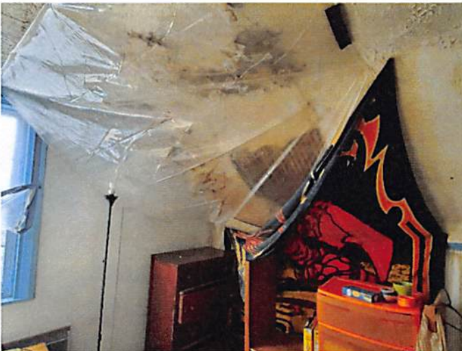
Collapsed ceiling in second floor bedroom with active water leak.
