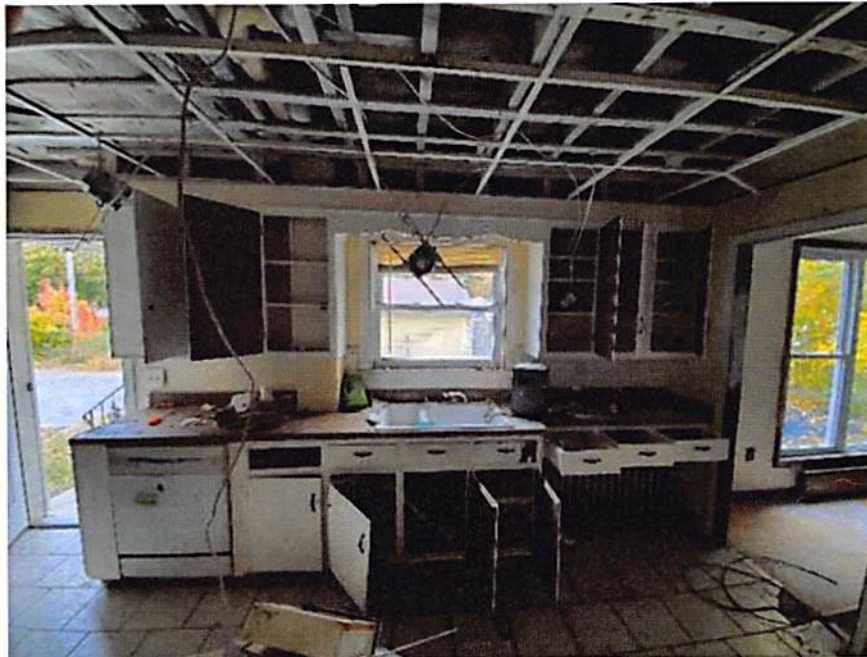
Missing ceiling, hanging electrical, missing/damaged plumbing, damaged structural elements
