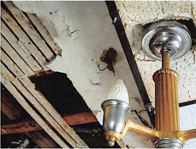
Collapsed ceiling in second floor bedroom with active water leak.
