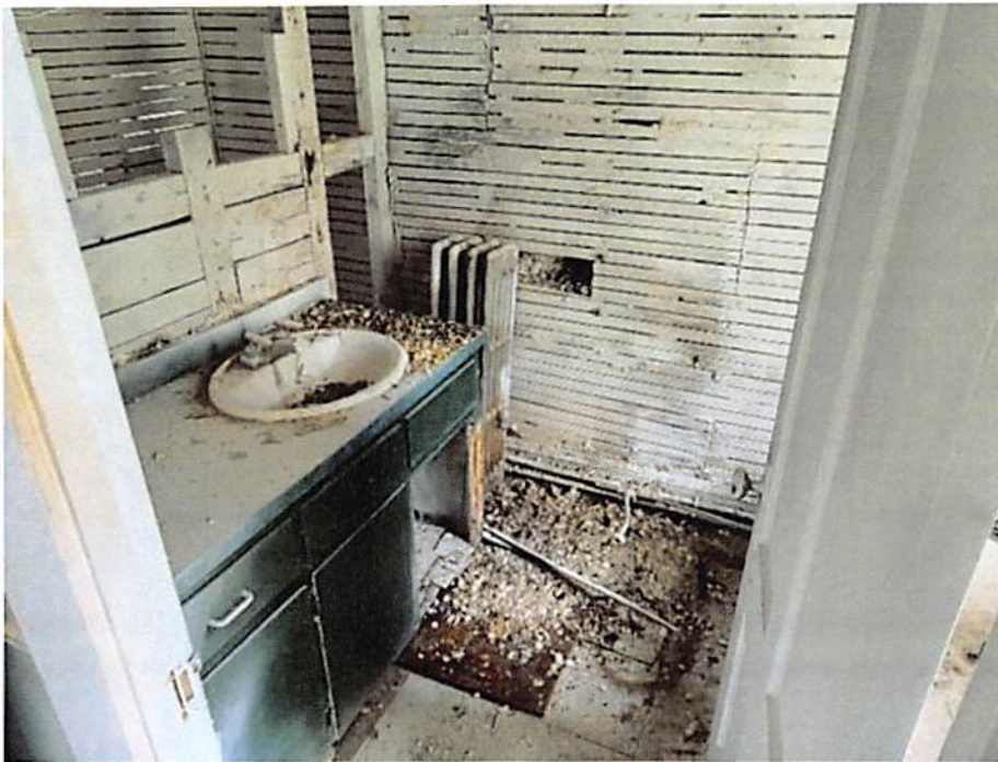
Deterioration caused by exterior elements and rodents Violation: Sec. 12-226. – Maintenance & Sec. 12-232. - Insect and rodent control.
