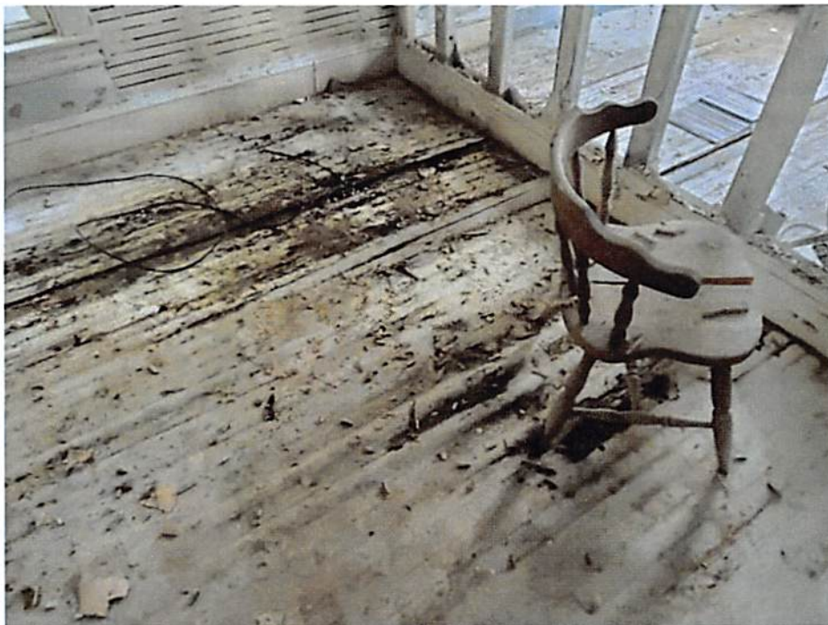
2 nd Floor deterioration (structural) due to exterior moisture intrusion Violation: Sec. 12-226. - Maintenance
