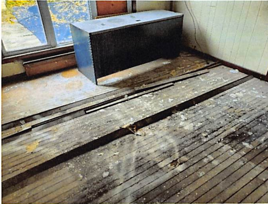
1 st floor deteriorated flooring to due exterior elements
