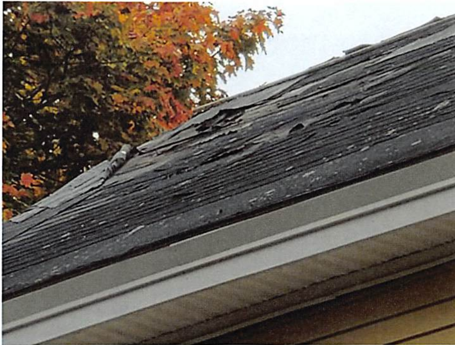
Continuation of roof deterioration Violation: Sec. 12-226. - Maintenance
