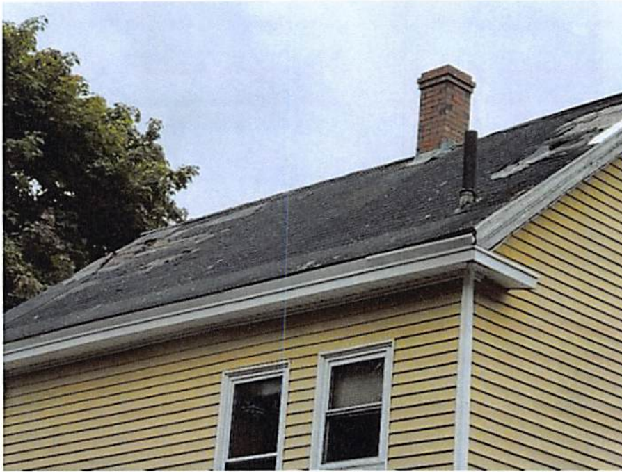
Holes and deterioration of the roof allowing the exterior elements inside
