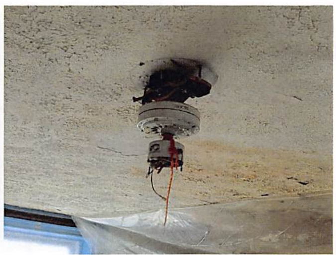
Broken light fixture with exposed wiring,
